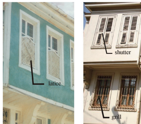
Fig.18. Generally, the Shutters, Lattices, Wood Railings or Iron Grills are Façade Characteristics of Wooden Houses
