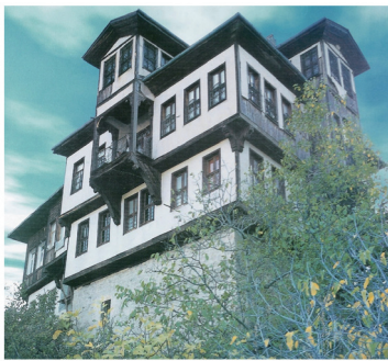
Fig.17. Roof Room Located in the Middle of the Roof
