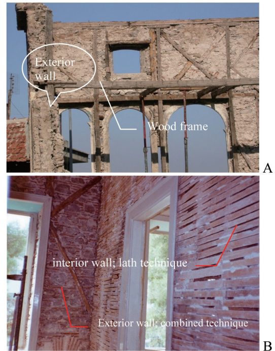
Fig.5. General View of Combined Construction, A: Kılıcı Mescid, B: Murat Residence, Izmir/Turkey (Photo by the Author)
