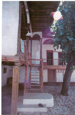
Fig.13. The Yard, Service Place and Stairs of a House in Muğla
