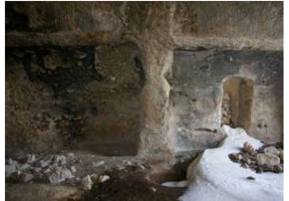
Fig. 46. Detail from stable in Area 14: The south of the large room on the exterior. Traces of mangers can be seen flanking the gate.
