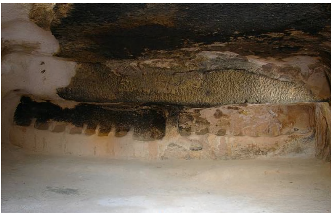
Fig. 23. Interior of the stable of Açık Saray No. 2a. View from the entrance towards the longest wall where the mangers are lined.
