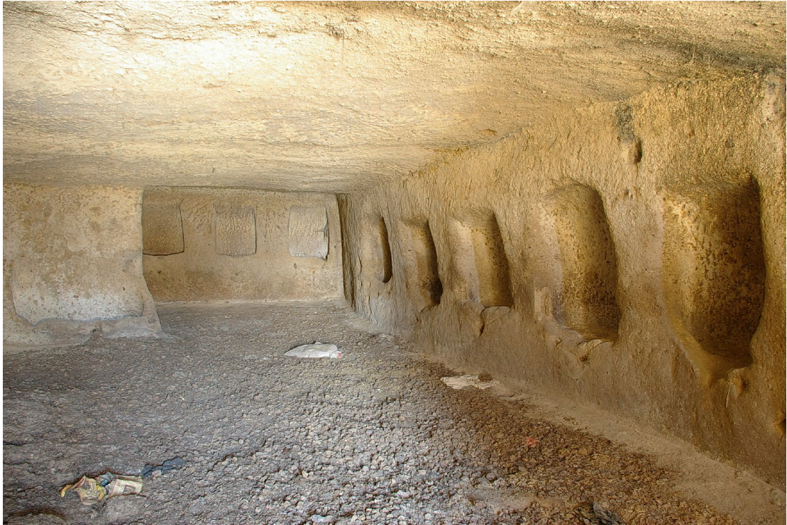
Fig. 18. A multi-functional stable in Selime with diverse sized-mangers. The mangers on the right are for cattle, height: 50 cm; the low ones on the left are for sheep and goats, height: 20-30 cm, the three mangers at the rear are for horses, height: 80 cm.
