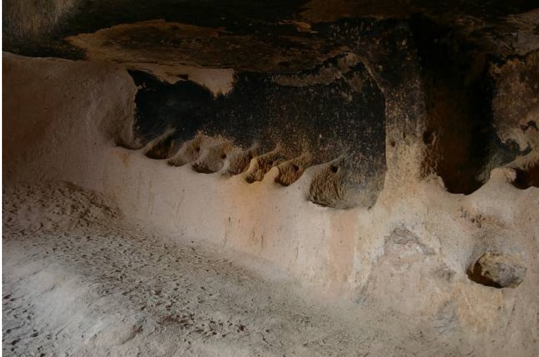
Fig. 24. Detail of mangers in the stable of Açık Saray No. 2a. The floor slopes towards the center to facilitate removal of droppings.
