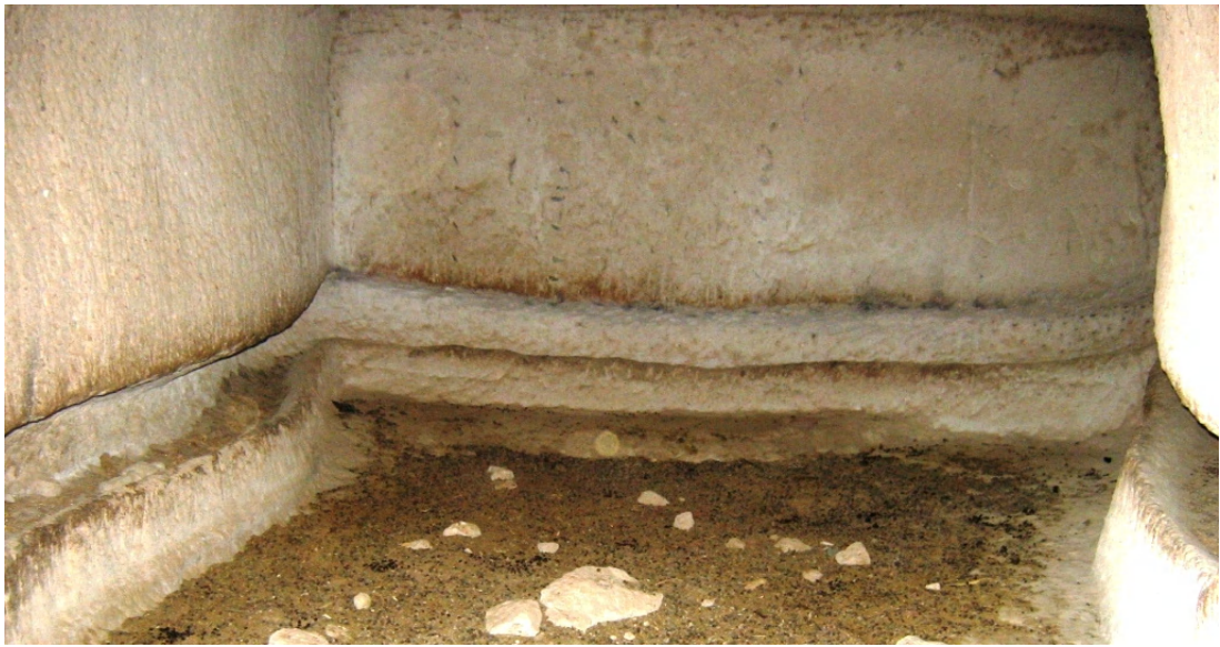
Fig. 8. Mangers for sheep and goats, height: 30 cm. Stable currently functioning in Selime.
