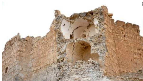
Figure 26. Collapse of a portion of northeastern wall (CNN; March 27, 2016)
