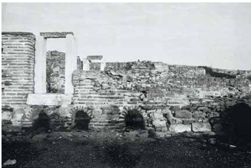
Fig. 76. The Baths ( Thermae ). The large complex of public baths at the southwest edge of the shrunken Roman and Early Byzantine city (TH on Map 18, p. 106).
