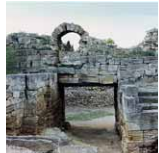
Fig. 185. In AD 488, when Emperor Zeno ordered the repair of the ancient walls, an arched entrance was built on top of the gate of the Hellenistic walls (dated in the 3rd-2nd c. BC).
