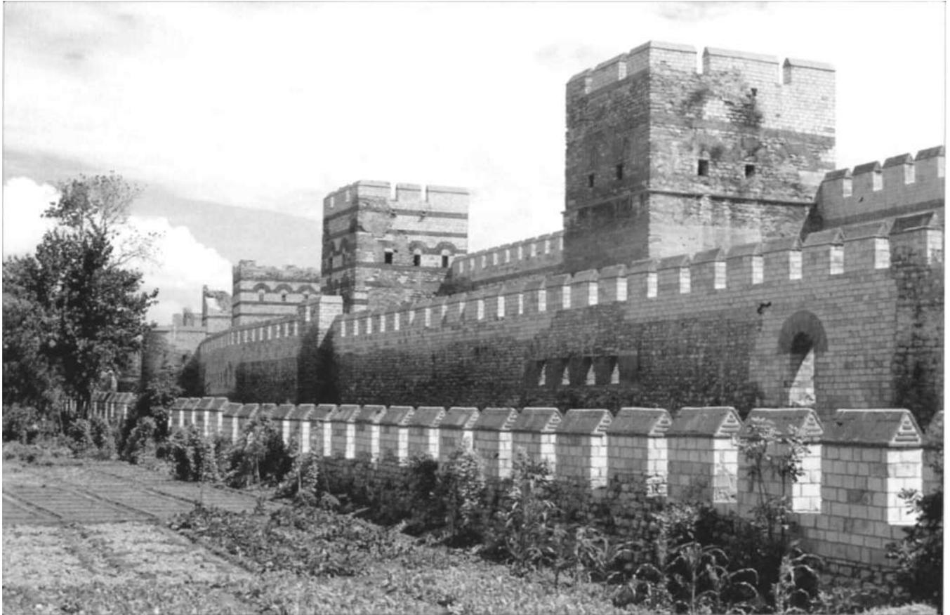
Possibly the finest restored section of the Theodosian walls lies here to the north of the Belgrade Gate. The complete system of inner wall, towers, *peribolos*, outer wall, outer walkway, small parapet and moat are shown here.
