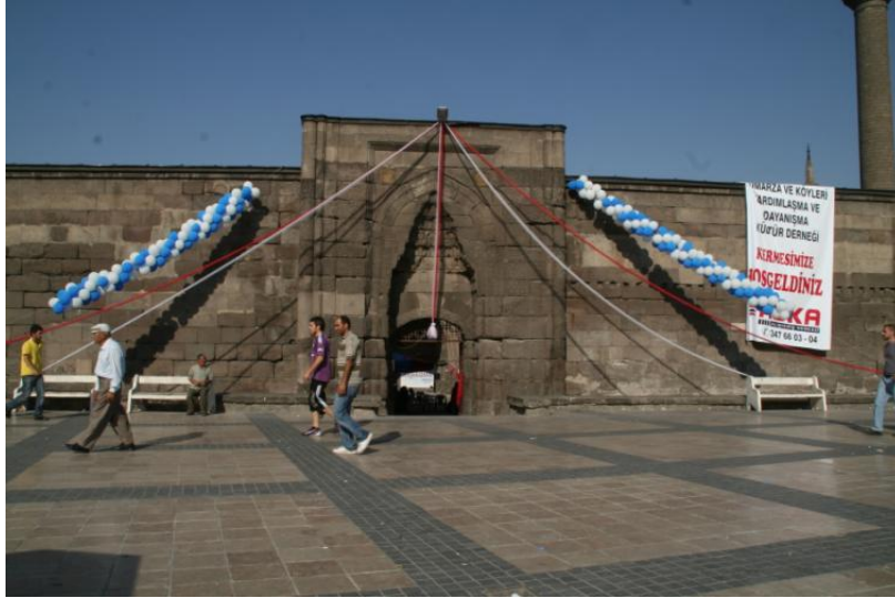
Figure 8: Huand Hatun Complex, Kayseri, portal of the madrasa (photo: author)
