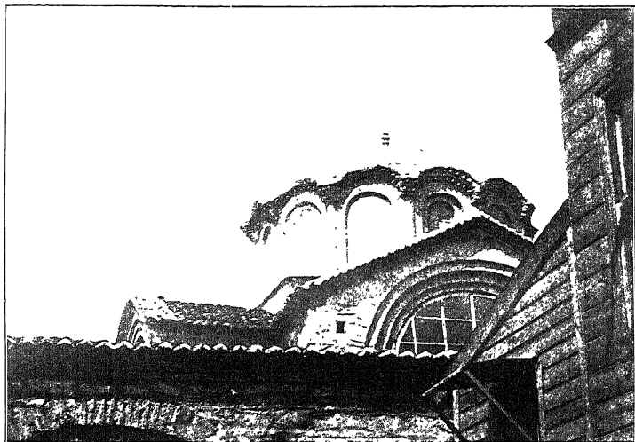
S. THEODORE. THE CENTRAL DOME, FROM THE SOUTH.
