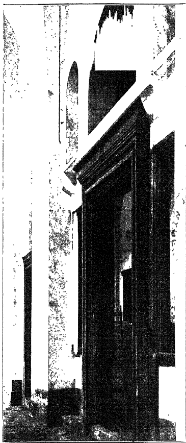
S. SAVIOUR PANTOKRATOR. ENTRANCE FROM THE NARTHEX TO THE SOUTH CHURCH.
