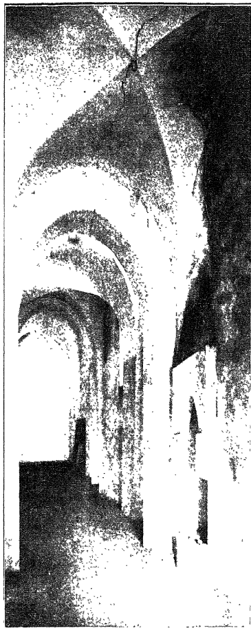
S. SAVIOUR PANTOKRATOR. GALLERY OF THE NORTH CHURCH, LOOKING SOUTH.
